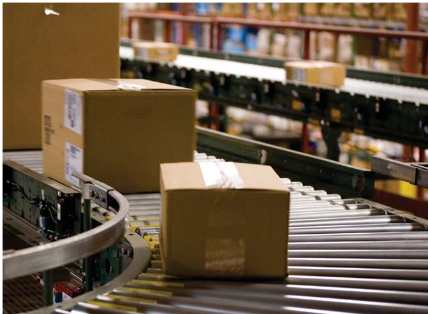
Logistic center and conveyer
